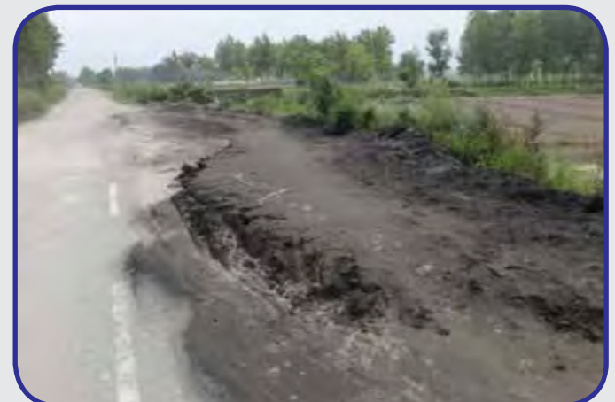
Disposal of RHA along road sides
